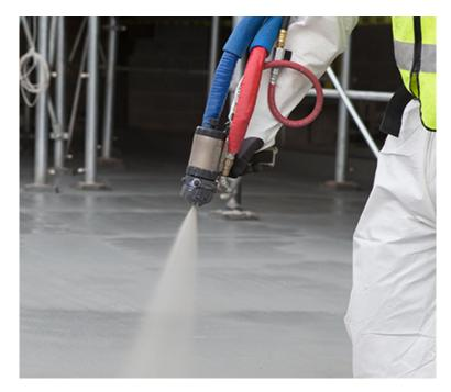
Prior to reconstruction, Tab Associates needed to find a weather barrier that would do the job. They needed the barrier to be seamless, to seal around fasteners, and be impermeable to liquid water. In addition, since the previous moisture barrier had been incorrectly installed by the original architect, Tab Associates wanted to find a product supported by technical services that would help them do the job right the first time.
