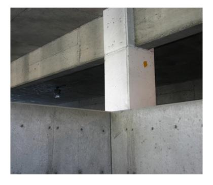
Carl Walker, Inc., the structural engineers for the project, were given the task of rapidly installing hard-wearing, crack-resistant concrete in high-traffic areas such as the slab-on-ground concrete, the pedestrian ramp and the loading docks. As the designers of over 1,000 multi-level parking facilities, they have successfully used STRUX®90/40 synthetic macro fibres in a number of previous jobs requiring fatigue resistance and high strength.
